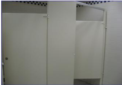
Men's bathroom, post clean up
